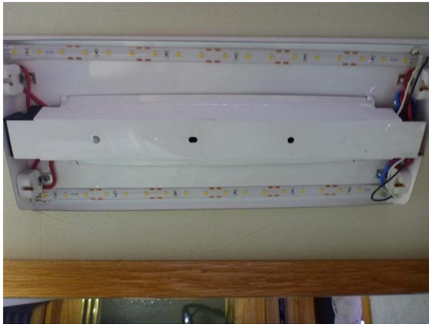
Center cover replaced over the wiring.
