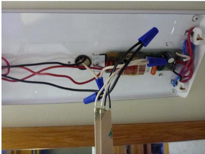
Connecting the LED strips to the power wires in the fixture.
