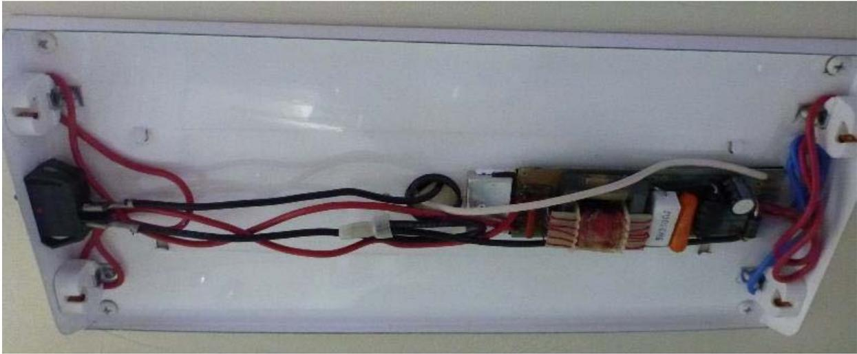
Squeeze and remove the cover over the ballast circuit and wiring.
